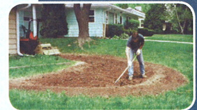
Rain garden under construction.
